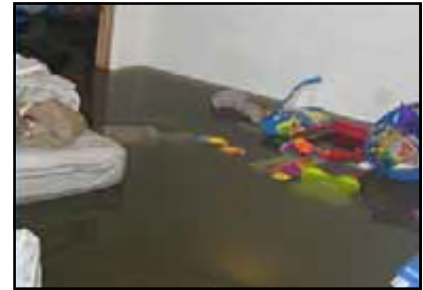
Sewer backup in residential basement.
